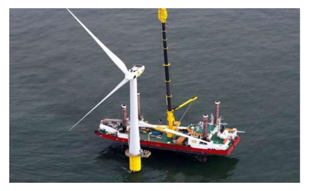
The Wind is a Jack-Up platform(Wind Farm Installation Vessel) measuring 55 metres in length and has a 4.3 metre draft, coloured Red and white. When jacked up the Wind will be marked and displaying lights and day symbols in accordance with an Offshore Structure.
