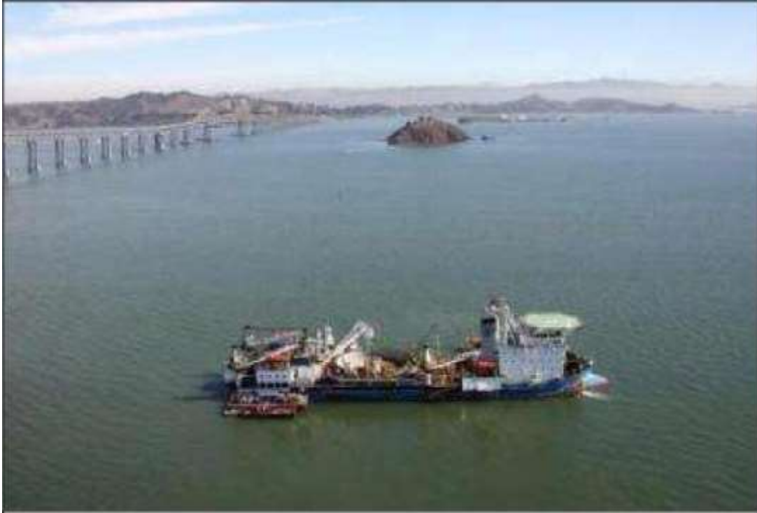
Cable Laying vessel - Giulio Verne
