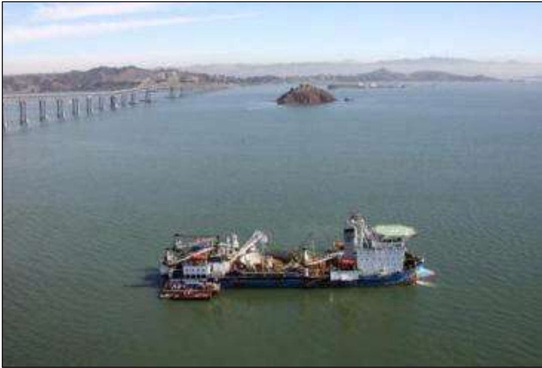
Cable Laying vessel - Giulio Verne
