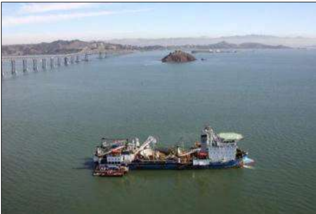
Cable Laying vessel - Giulio Verne
