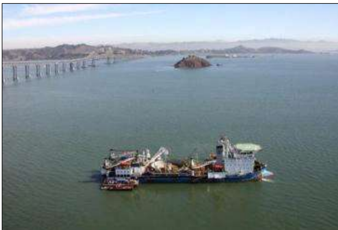
Cable Laying vessel - Giulio Verne
